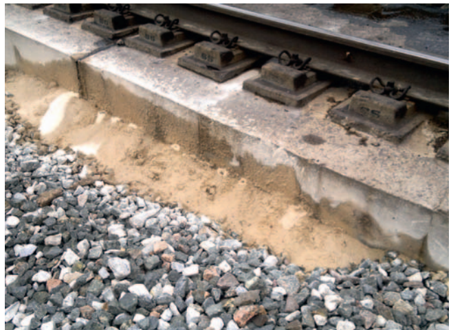
Fig. 5. Pumping from under the structural slab (Tines)
