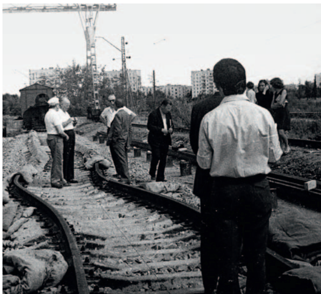
Track buckling tests
