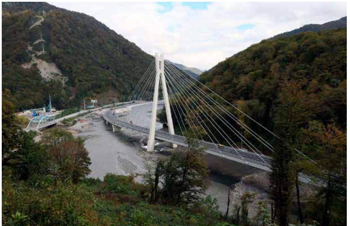
Fig. 2. Cable bridge span on the Mzymta River
